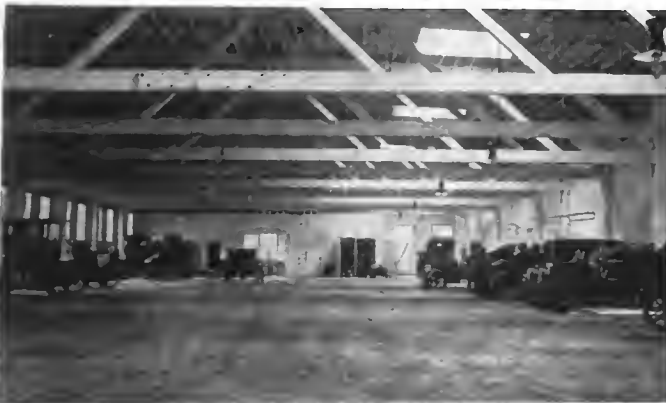
INTERIOR NEW GARAGE ATWOOD AUTOMOBILE CO., TOLEDO, O.
